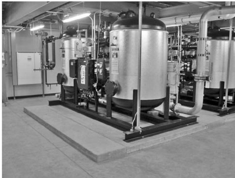
FIGURE C13.1-7 Skid-Mounted Components
