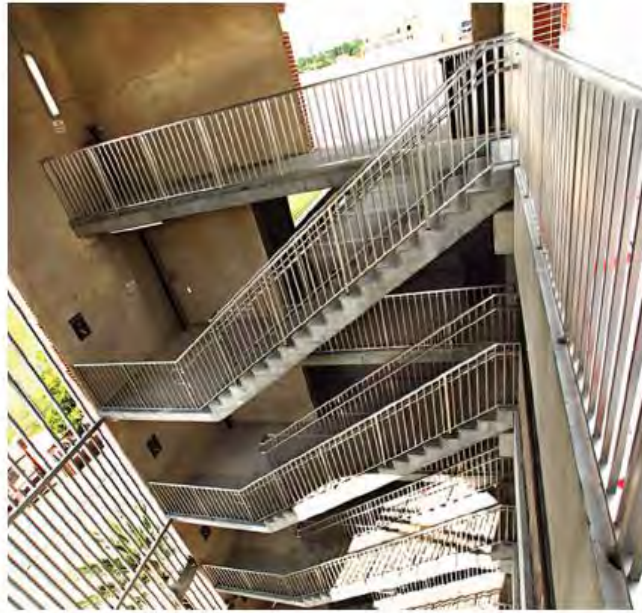
FIGURE C13.5-2 Steel-Framed Exit Stair
