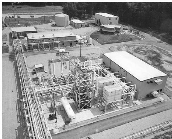
FIGURE C15.1-2 Steel pipe rack
