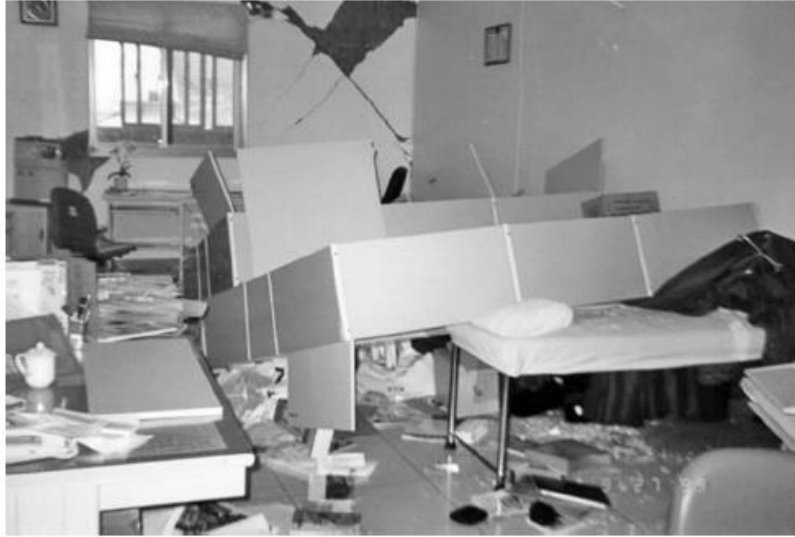
FIGURE C13.1-4 Toppled Storage Cabinets
