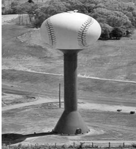
FIGURE C15.7-2 Small-diameter, single-pedestal steel tank
