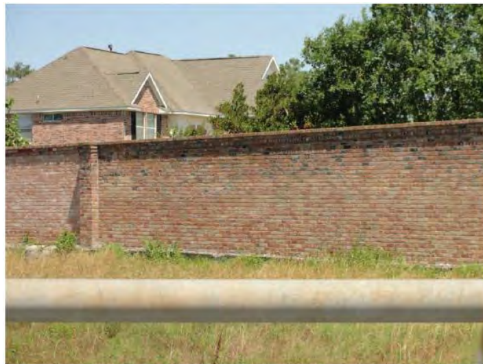
FIGURE C15.6-4 Typical Masonry Ground-Supported Cantilever Wall
